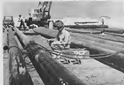
A SHARP tool, above, means a sharp job, and this worker tends his tools on the Oranjestad terminal project. A welder, below, prepares pipe before it is laid in trenches. UN HERMENT skerpi, arriba, ta nifica un trabao delcado, y e trahador aki ta manehando su hermentnan. Un welder, abao, ta prepara tubo promer cu hinea nan den e zanja.
